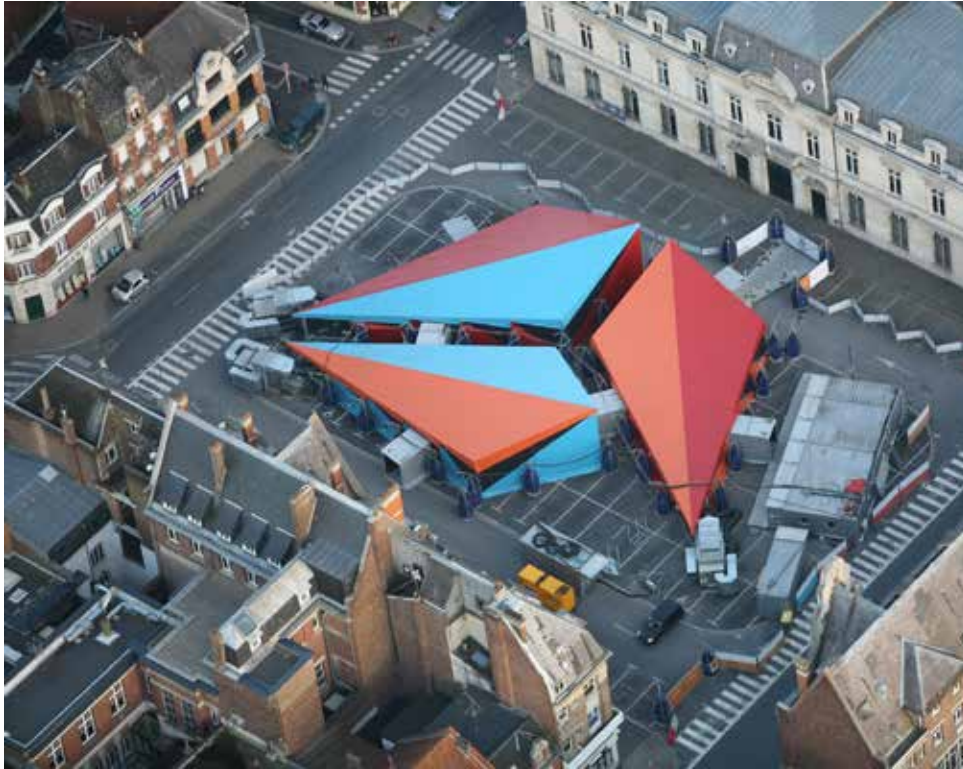
Centre Pompidou Mobile, Cambrai - Construire Architects, photography Studio Déclic, February 2012
